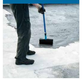
V-Flex G2K is a two-component cementitious polymer modified elastomeric, waterproofing & protective coating, which reduces the room temperature up to  $7 - 9^{\circ}$ C at peak summer hours.
