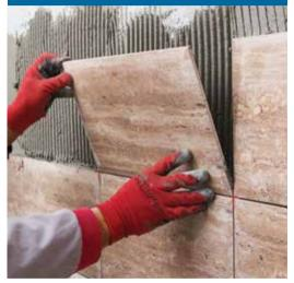
Reve Fix is a polymer modified, cement-based, pre-packed and ready to use tile adhesive.
